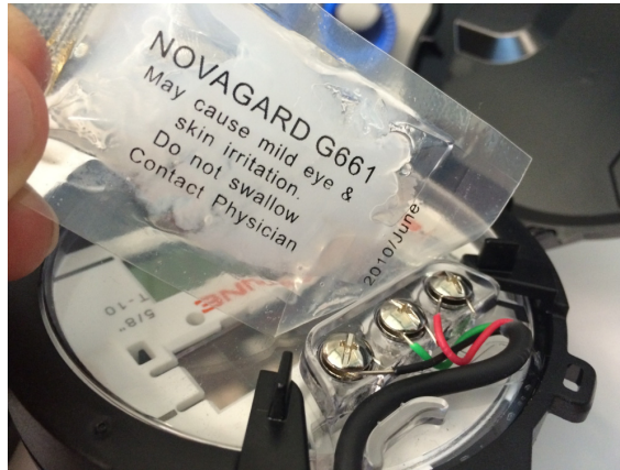
Figure 11 Application of the Sealant
