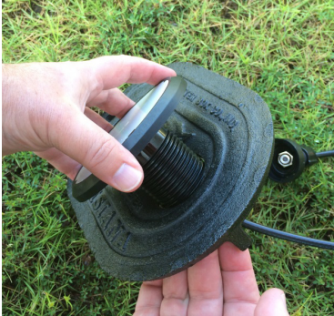
Figure 26 Inserting Antenna into the Pit Lid
