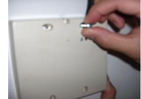
**Step 4:** Identify the outer half of the IREP enclosure. Secure this half over the first half using the  $#6-32 \times 1''$  button-head screw (E) at the top center of the IREP.
