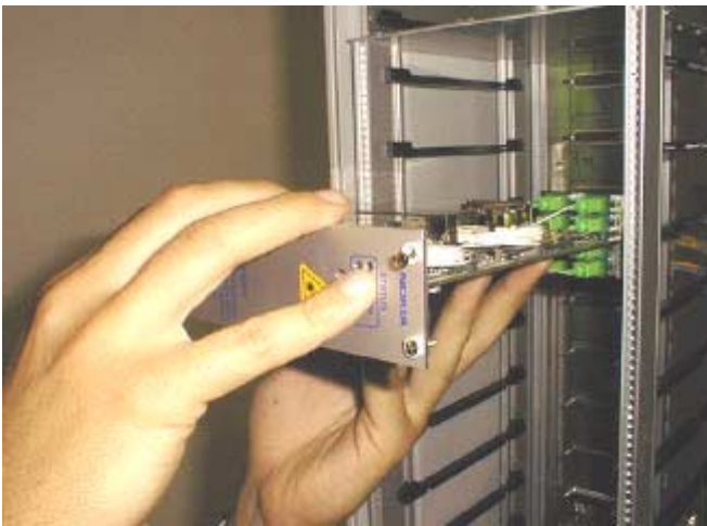
Figure 2 Installing the LU
