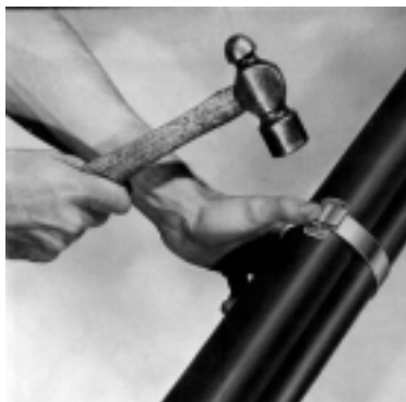
Fig. 3.14. Hammering buckle ears
