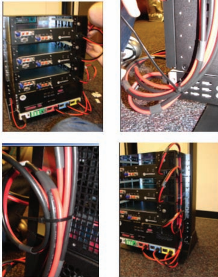
Figure 3-11 Tying power cables to the cable tie brackets
