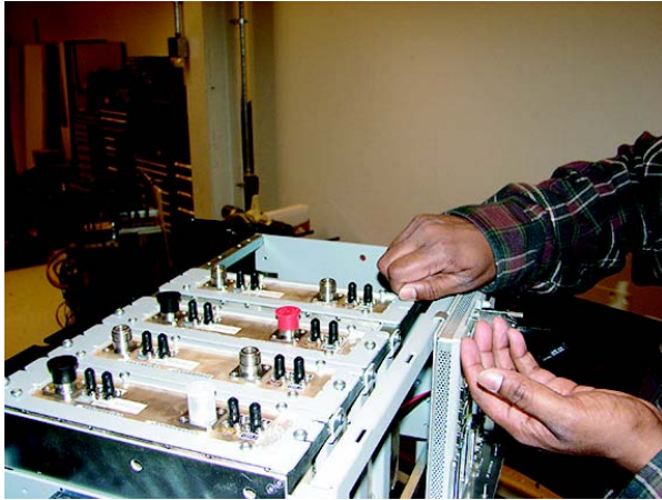
Figure 3-4 Installing the second set of IDRFs
