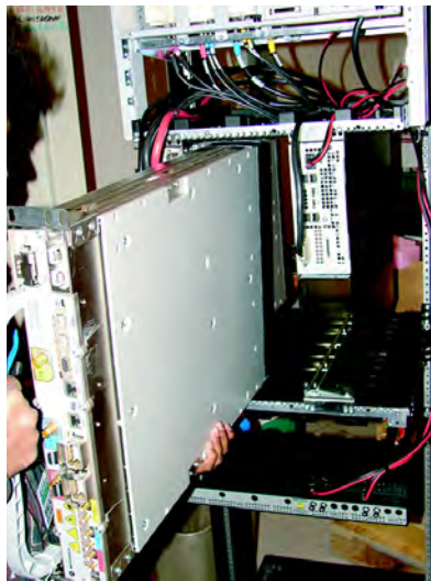
Figure 3-2 Installing a 2nd XMI
