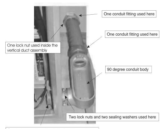
One lock nut and one insulating bushing used here
