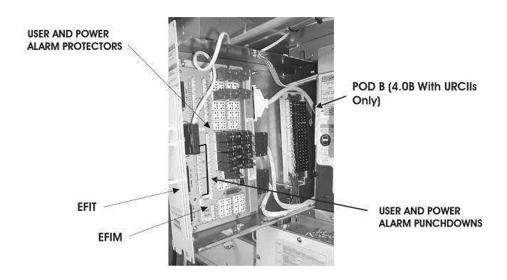
**3** Connect the alarm wire pairs. Refer to the figure on Page B - 38 and the table on Page B - 39. Start at pair 0 (zero).
