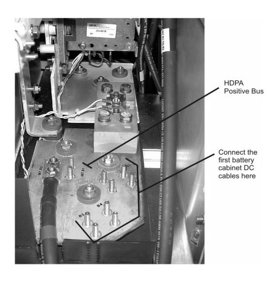
Connect (or reconnect) the 24V Return cables from the first battery base module to the return bus in the Modular Cell 4.0B cabinet Perform the following steps to connect (or reconnect) the four 24V Return cables from the first battery base module to the return bus in the Modular Cell 4.0B cabinet
