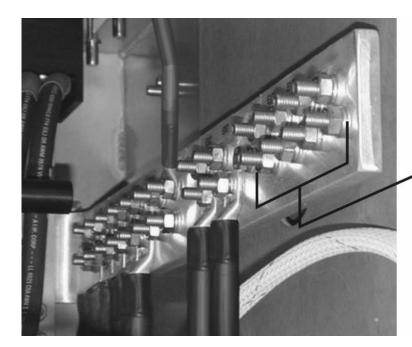
Connect or reconnect four 24-VDC return wires from battery cabinet here
