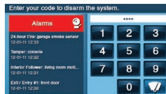
Disarm Screen Showing Alarms
