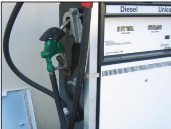
Figure 1-1. Regular NR Installed on Pump
