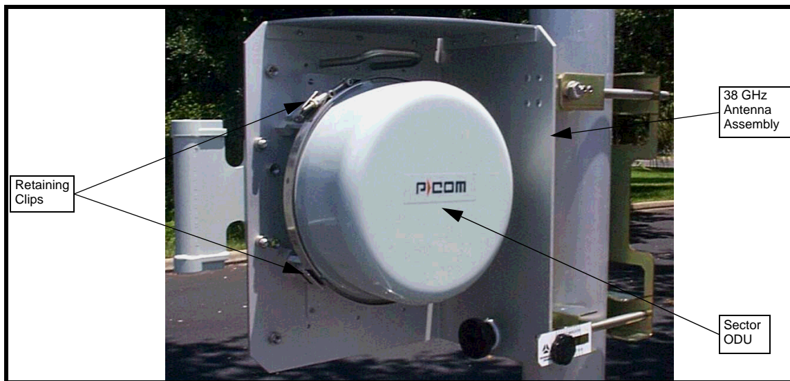
Figure 6-8 - Attaching 38 GHz ODU to Antenna Mount Assembly
