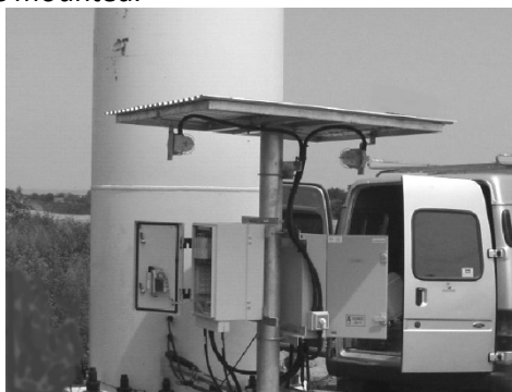
Figure 4-3: Example of a sun shield Repeater Installation
