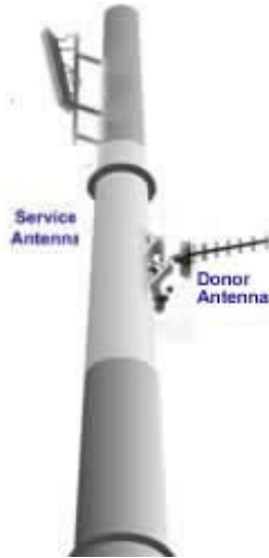
Figure 2-1. Service above Donor Antenna
