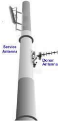
Figure 2-3. Service above Donor Antenna
