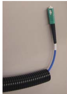
Figure 2-18: Run Optic Fibres through Sleeve
