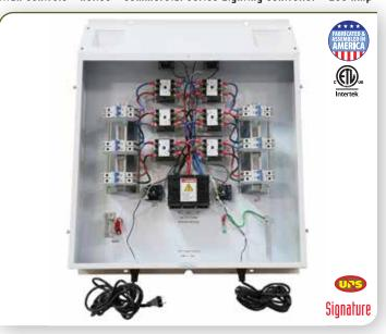
The Commercial Series 200 Amp Lighting Controller features: Allen-Bradley ballast rated industrial relays, Allen Bradley 30 Amp circuit breakers, dual trigger cord sets to activate lights, 0-30 second timing modules to delay HID bulb strikes. Comes with a three phase wiring configuration. It features a 20 gauge powder coated steel panel, convenient side wiring knock-outs, top power exit ports with knock-outs and manufactured in the USA. Commercial Series panels are built to be Titan tough!
