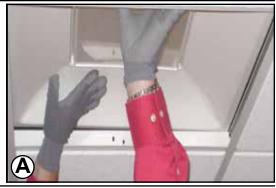
Step **⑤**: Remove wire-way cover and remove appropriate knockout to route input conduit. Connect wires as shown in wiring diagram. Push all wires back into wire-way and replace cover. (see Detail B).
