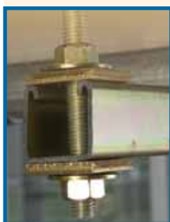
Standard method using nuts and washers
