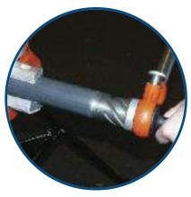
$Ream\ the\ conduit\ with\ approved\ reamers.\ Spiral\ and\ straight-style\ reamers\ are\ both\ acceptable.$
