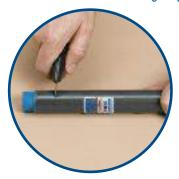
Step 2 calls for the edge of the PVC that was cut on the perpendicular to be carefully lifted to form a plastic tab.
