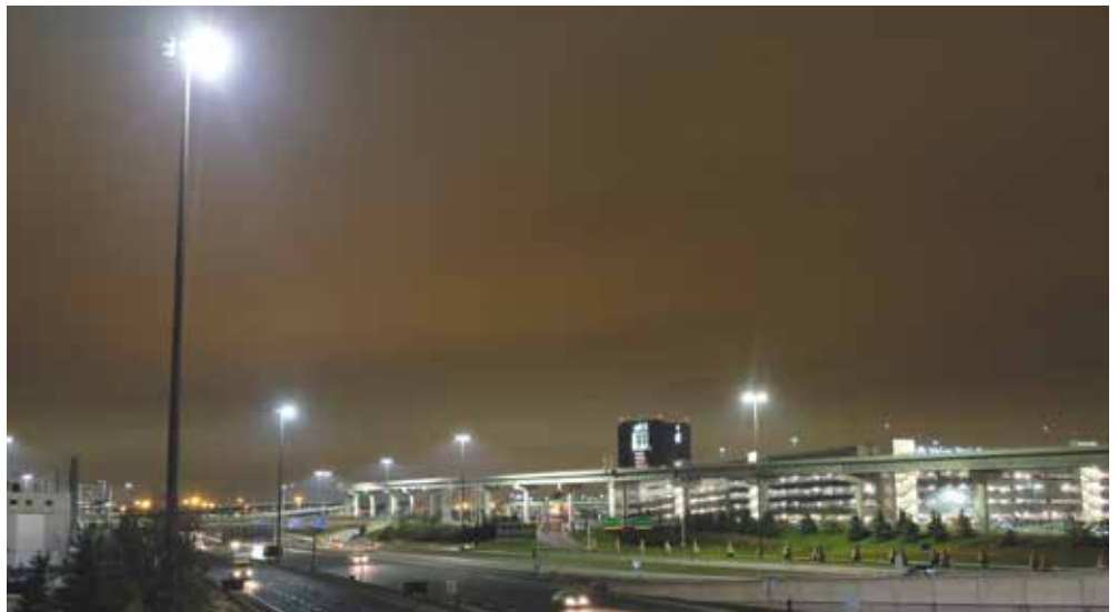
▲ Night-time driving along the 409 in Toronto is now a little different thanks to some changes with the high-masts. PHOTO COURTESY GTAA.
