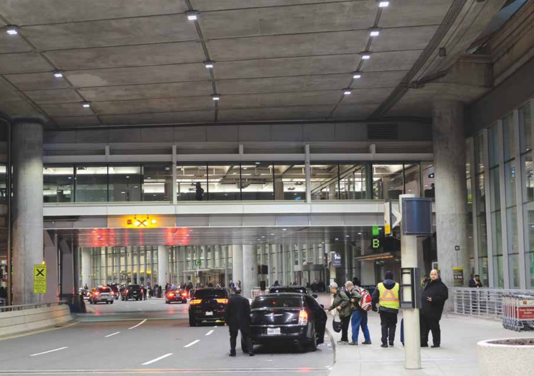
▲ The Arrivals platform at Terminal 1 is newly bedecked with LEDs emitting 7000 lumens each. PHOTO COURTESY GTAA.
