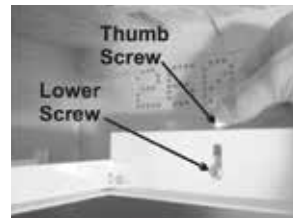
5. Tighten lower screw to adjustable bracket to make flange kit flush with ceiling surface. Next, tighten thumb screw to secure into place.
