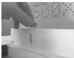
3. Gently tighten thumb screws ensuring adjustable bracket is pressed lightly against drywall. Make sure NOT to tighten all the way.
