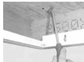
6. Install safety chain (by others) from holes provided on the top of side flange assembly to the ceiling structure.
