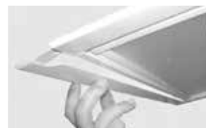
8. Slide in end flange trim (If row mounted then only required at start and end of run).
