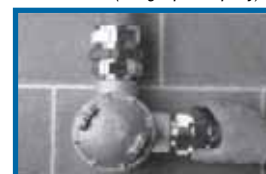
6. Insert cable and tighten red union
