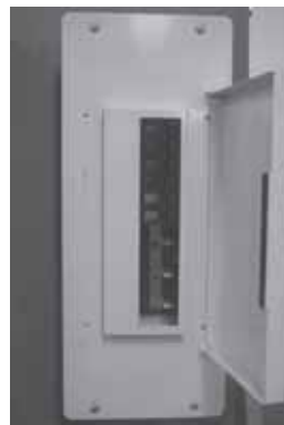
Step #3 Install New HFLCI
