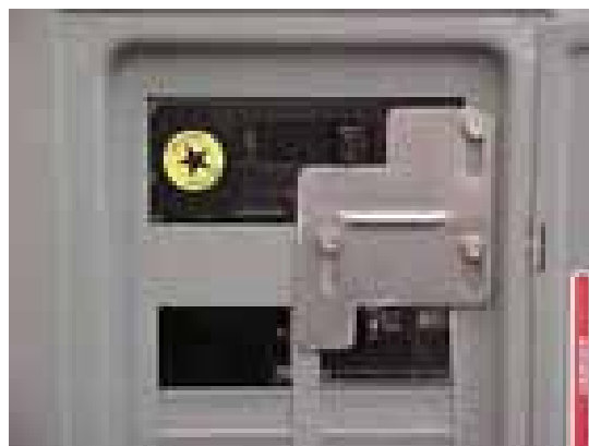
Generator Interlock Kit (In use)
