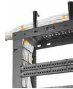
Wire Gates Installed
