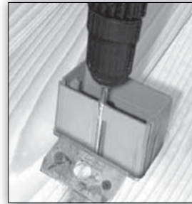
Screw In To Adjust To Height Of Flooring Or Carpet
