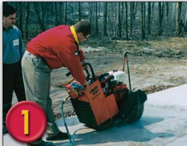
1 3/4" Sawcut The Pavement
