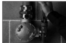
5. Install hub on enclosure
