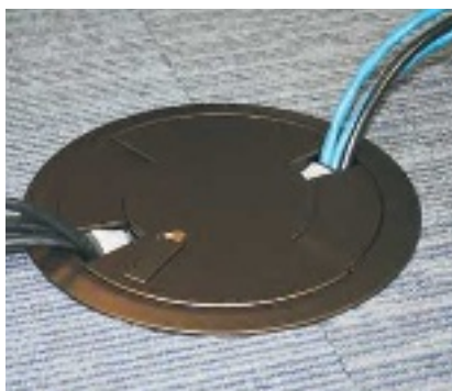
Cables egress from a CRFB Series Floor Box with Evolution Series Poke-Thru Cover.
