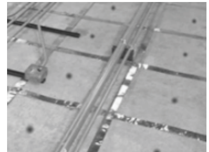
Pedestal locations marked by the dot
