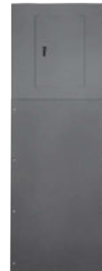
Panel skirt completely installed.
