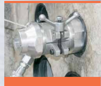
Complete the assembly and blow in tape.
