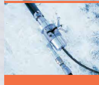
Complete the assembly, attach compressed air hose and blow in winch line.
