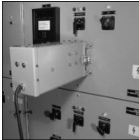
Figure 7 Motor drive mounted on CB cubicle door.
