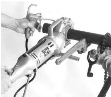
Threading using a pipe wrench as a support arm.
