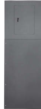
Panel skirt completely installed.
