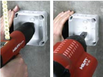
HILTI nailers are particularly adapted to fixing MUREVA boxes.
