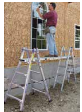
POSITION #4 Self-Supporting 2-Scaffold
