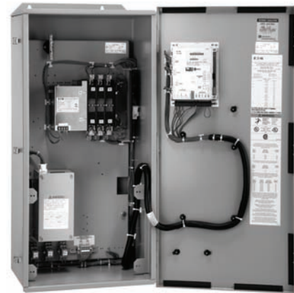
200A ATS with ATC-300 Controller
