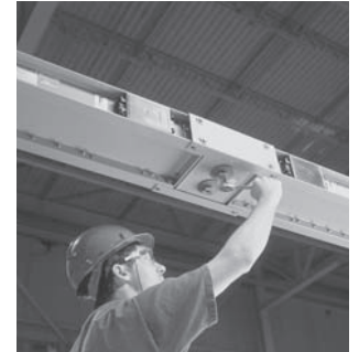
Typical Busway Installation (Torque Indicating Bolt)
