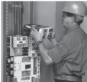
Panelboard Installation
