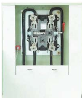
Bypass Section—Test Block
