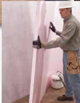
Easy foam board installation above or below grade
