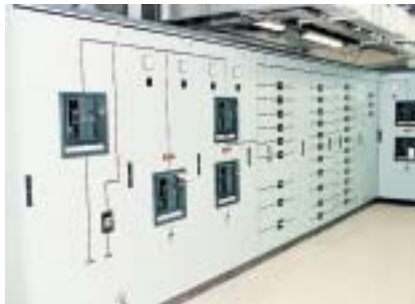
The main feature of OLN cubicles is that they can be joined together to form large bay switchboards and their full accessibility.
