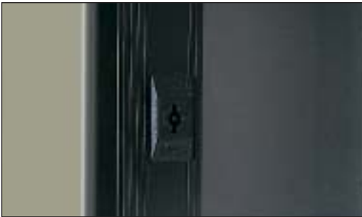
Detail of standard double bar lock fitted right on the profile for an excellent finish.
