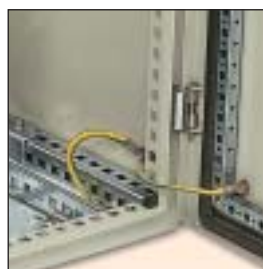
A complete system to earth the enclosure and components.
