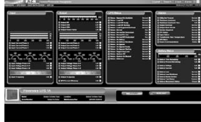
Eaton Powerware UPS-Primary View
