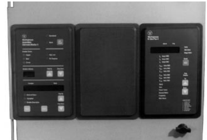
DS Replacement Door with AEMII, IQ Data PlusII, Poni Cards (2), and Blank Plate
