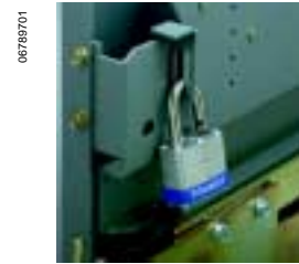
Padlocked Drawout Carriage Hasp
