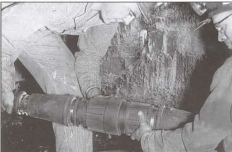
Quik-Loc Connectors fully engage or disengage in only 3/4 turn of coupling. Largest will handle up to 500 MCM cable.
