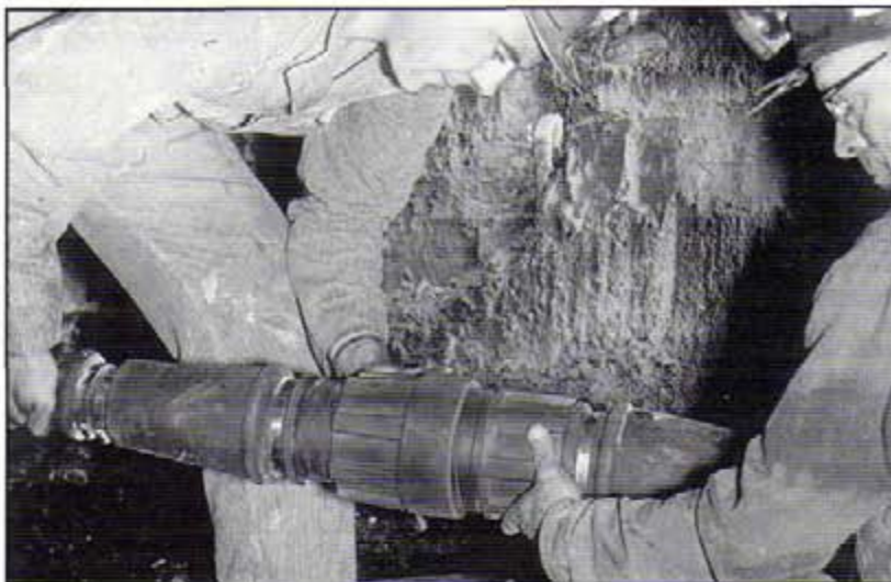
Quik-Loc Connectors fully engage or disengage in only 3/4 turn of coupling. Largest will handle up to 500 MCM cable.
