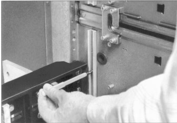
3.) Install four (4) Shutter Rails (2 per each side).
