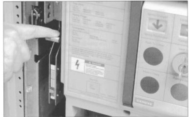
Interlock Lever mechanism
