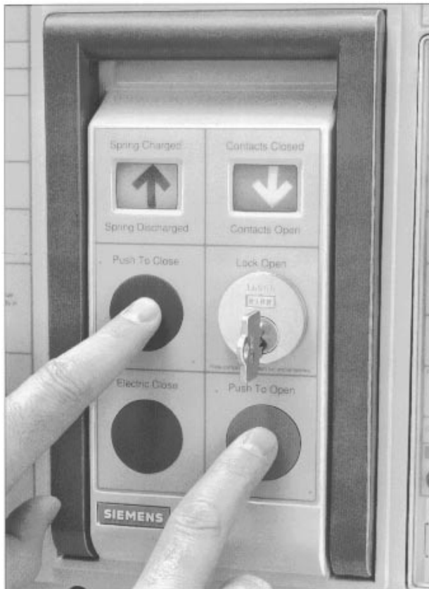
Discharging energy in the stored energy mechanism
