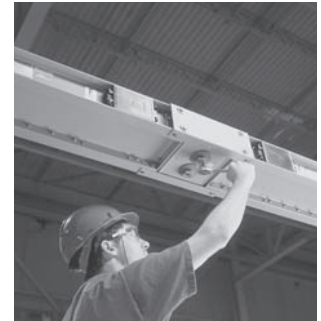
Typical Busway Installation (Torque Indicating Bolt)
