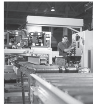
Final Busway Assembly
