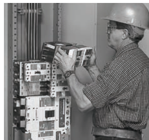
Panelboard Installation
