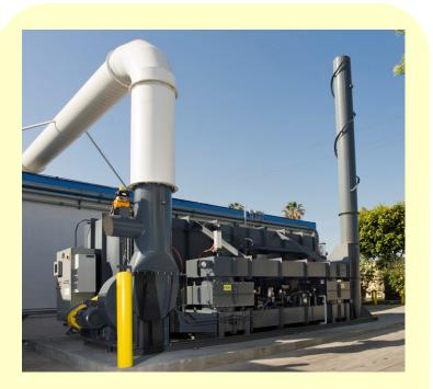
Our California facility takes pride in limiting volatile organic compound (VOC) emissions into the environment. Two regenerative thermo oxidizers are utilized to eliminate 99% of the VOC from our ventilation system before emitting air into the atmosphere.
