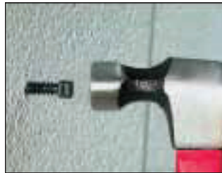
2. Hammer mount into hole.
