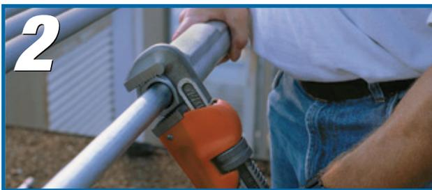
With a wrench, tighten the gland nut to compress the Teflon packing, creating a raintight seal around the conduit.
