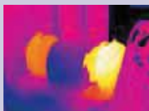
Overheating bearing cap
